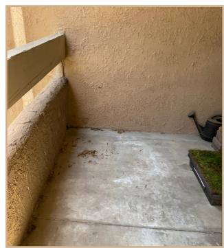
The concrete walking surface and stucco assembly show no signs of water intrusion or building component failures.
