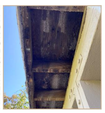
Based on results from the borescope investigation, we removed soffit materials and the extent of the concealed damage is very apparent.
