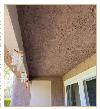
The underside (stucco soffit) showed no visual signs of water intrusion into this soffit
